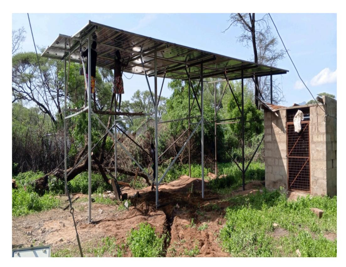
Fully installed and equipped solar plant at the lopiding borehole that provides energy for pumping water from the borehole.
