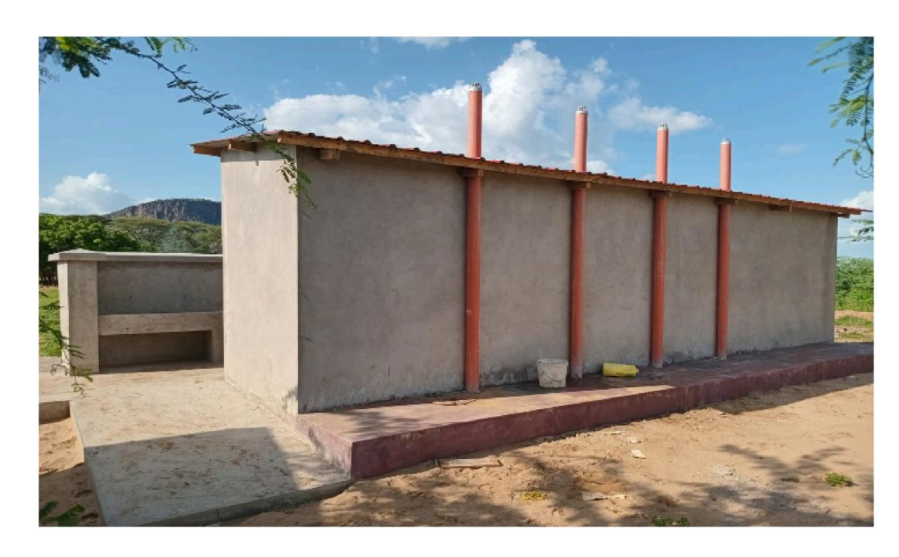
The back side of a school VIP latrine featuring the manholes which will allow for emptying of waste once the pits fill up.
