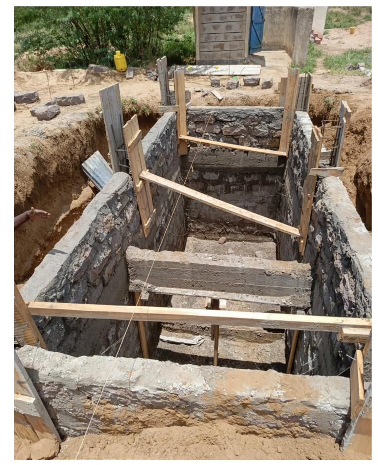
Pit lining to avoid collapsing due to loose soils
